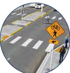
**Pedestrian refuge islands** provide protected spaces midway across the roadway for pedestrian to safely wait in and are useful where a long crossing cannot be sufficiently shortened using corner bulges and curb extensions.
