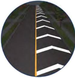
**Transverse pavement markings** are a series of white transverse bars that are spaced across the center of a lane to create an illusion to drivers that they are increasing their speed.
