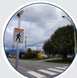
**Pedestrian activated flashers** warn drivers to slow down and stop for pedestrians crossing when activated by a push-button.
